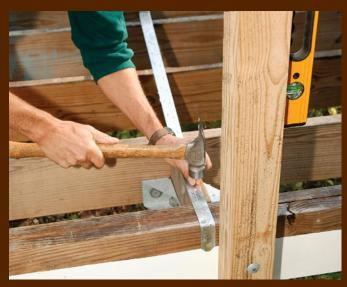
Use a strap to reduce wobble. If you bolt on posts at the framing stage, you'll notice that the posts on parallel rim joists will have a lot more deflection than those along perpendicular joists. Once the decking is installed, the deflection diminishes. Go one step further to help stiffen these posts by nailing a 16-ga. metal strap across the top of the rim joist and the next three or four inboard joists.
