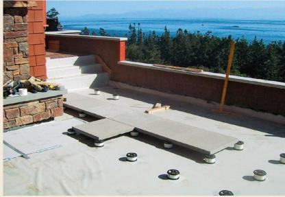
**Level pavers on a sloped deck.** Concrete pavers atop a Duro-Last membrane compose the finished walking surface at the entry court. The pavers are supported at their corners by pedestals that consist of a base, a cap, and a piece of 4-in. plastic sewer pipe (www.appianway system.com). Each row of pipes gets a little taller as it moves down the slope so that the pavers end up level. A PVC slip sheet under each pedestal protects the membrane.
