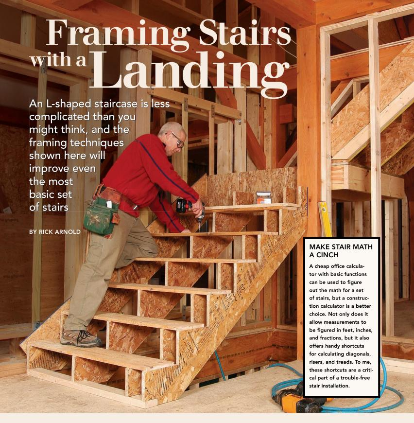
hen builders struggle with a stair layout, it's almost always because they get hung up on the rise portion of the calculation, especially with the adjustments for flooring and stair treads that haven't been installed yet.
