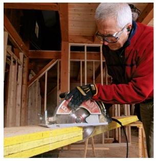
The marked stringer becomes the template. With the marked stringer on top, clamp all three pieces together, and gang-cut them using a 10-in. circular saw (www.bigfootsaws .com). Don't overcut the inside corners of the stringers; finish the cuts with a reciprocating saw instead. Last, trim the plumb cut of the middle stringer by 1/8 in. to set it back slightly when installed. This eliminates the chance of bowed finished risers.
