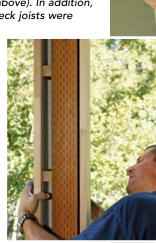
back of the trim with lineman's pliers to avoid blowouts on the finished side of the wood, then scraped off the multiple coats of paint that had accumulated over the years. One column was too badly cracked to repair, so I replaced it with one I made from primed red cedar that will probably outlive the rest of the porch.
