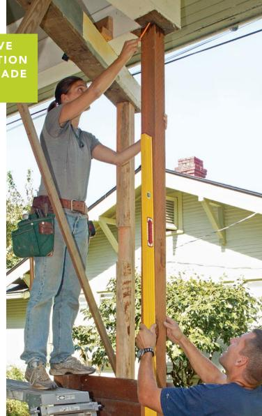
remove the old structure, and pour adequate footings. In the end, I also rebuilt the enclosed railing walls.
