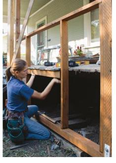
**Tend to the frame first.** After the new posts were installed, the enclosed railing wall was reframed with new pressuretreated lumber (photo above). In addition, any rotted or suspect deck joists were
