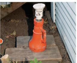
Jacks need a solid base. Jacks are positioned under each end of the carrying beam. Because soil conditions vary from site to site, it's important to choose a base that can support the load of the jack and keep it from sinking or tipping over. Soft soils require a wide base. Here, a pair of 4x6 blocks was sufficient to form a stable base.
