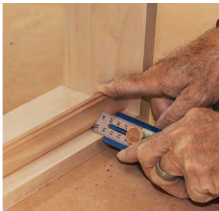
Stop centers the sash. To center the transom sash in the jamb, nail the sash stop molding \frac{3}{4} in. from the edge of the jamb.
