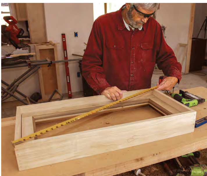
Stop centers the sash. To center the transom sash in the jamb, nail the sash stop molding \frac{3}{4} in. from the edge of the jamb.
