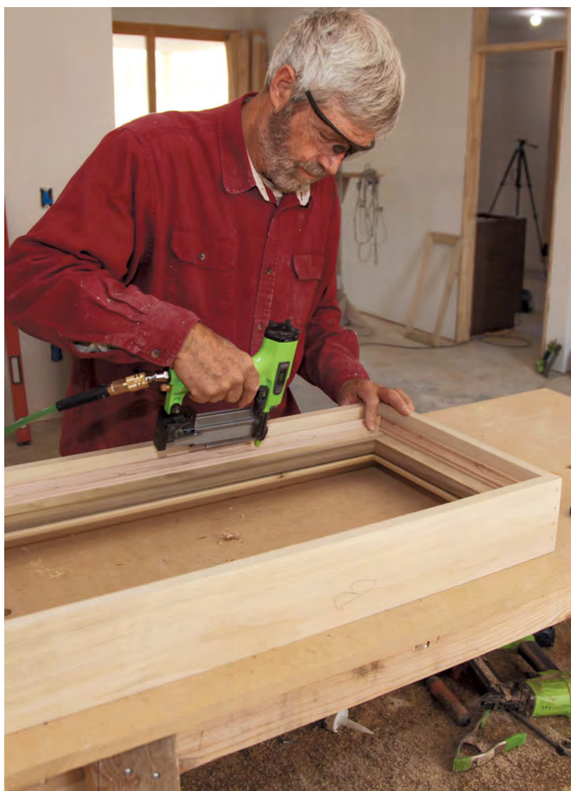
Second stop holds the sash. With the jamb square and the sash tacked in place, apply the inside bead of sash stop to permanently secure the sash in the jamb.
