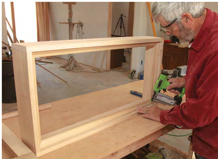
Stop centers the sash. To center the transom sash in the jamb, nail the sash stop molding \frac{3}{4} in. from the edge of the jamb.
