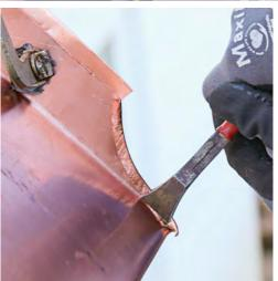
**TIGHTEN THE CURVES** At the bottom of the roof, a curved steel dollie provides enough mass to keep the seam upright while the longer rib is folded over the shorter one. We pinch the seam fully closed using special pliers.
