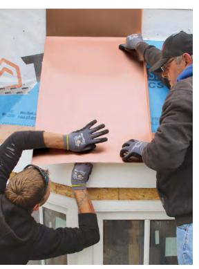
MARK THE HEM With the first panel's right edge aligned to the centerline of the roof facet, we scribe the roof edge on the bottom of the panels and then add 1 in. for the hem on the bottom of the panel that will later lock onto the drip edge.
