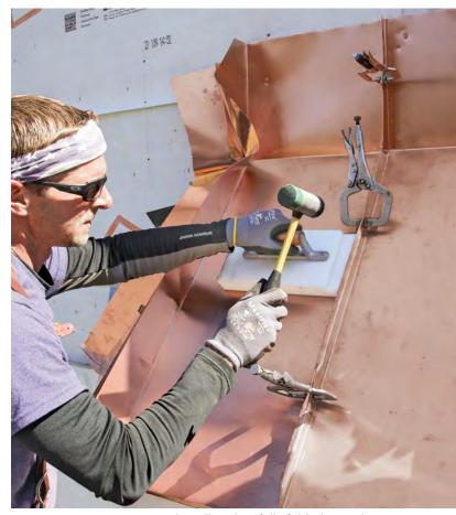
MAKE IT A DOUBLE Once the taller rib is fully folded over the shorter one and pounded flat along its entire length, the seam is folded a second time for the double-lock. Using the seaming tool's 1-in. notch, we pound over the seam, first 90° from vertical and then 180°, fully flattening the ribs for a second time and creating the double lock.
