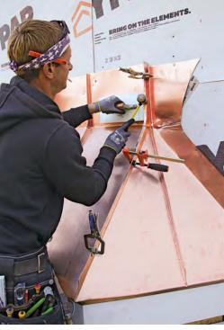
WORK YOUR WAY UP We work upward with the seaming block to create the first lock. At the pocket folds we flatten the seam above and below before flattening the pocket fold.
