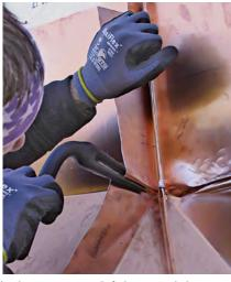
FOLD THE HIP POCKETS The pocket folds at the hip seams are left long until they are fully tightened; the extra copper provides grip for the fork and the additional surface area prevents tearing the copper. Once the folds are tightened with the forked tool, they're ready for trimming.
