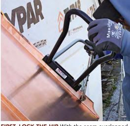
FIRST, LOCK THE HIP With the seam overlapped and folded, we pinch it fully closed using a seaming tool. This step helps straighten the seam, making it easier to accomplish the first lock.
