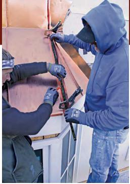
MARK THE TOPS We mark a 13/8-in. rib on one side of the hip seam with the panels clamped together and held tight to the roof. Then we trim the rib, moving the clamps as needed.
