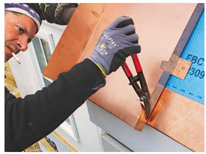
CUT THE CURVE One of signature details we learned from Joe Jenkins in a one-day course on traditional copper roof details is how to make a sloping curve at the ends of the ribs. We make a template that suits the height of the seams and scale of the roof and use it for marking the ends of the seams for cutting.
