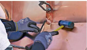
**POCKET FOLDS CHANGE PLANES** Where the roof panels meet the wall and where the kickout flashing projects we make pocket folds with a forked tool. After the pocket folds are tightened and trimmed, we pound the thick folds flat with a hammer and a steel dollie before following up with the PVC seamer.
