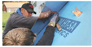
MARK AND BEND THE HIP With the side panel held on the roof, we scribe the location of the hip onto the back side of the panel.
