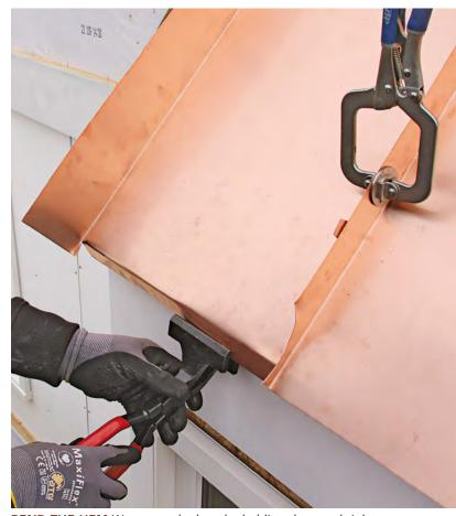
**BEND THE HEM** We create the hem by holding the panel tight to the roof and, through a series of about six smaller downward bends, we fold the hem over so it tightly grips the drip edge, working from one side to the other. Locking pliers for pocket-hole joinery are great for holding panels during hemming, forming, and seaming.
