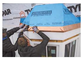
CUT AND BEND THE CENTER RIB The coil is cut to the length of the roof plane plus 10 in. to allow for the bottom hem and the roof-to-wall flashing. We form two panels with a bend at the top where they meet the wall and a rib on one edge—a 1¾-in. rib on one panel, which will be bent over the 1¾-in. rib on the other.
