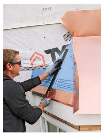
FIND THE CENTER The center seam where the pairs of side panels meet should be located in the center of the side roof facet for the best finished look. We mark the center on the drip edge and continue the line up the roof using a framing square. The panels edges are aligned to the mark.
