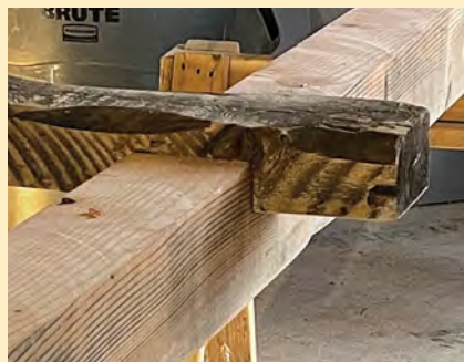
SQUARE SHOULDERS Cutting the mortises begins with circular-saw cuts across the beam to the depth of the joist tenons. A rafter square guides the cut to ensure the shoulders of the mortise are perfectly square. Additional cuts between the shoulders help with waste removal.
