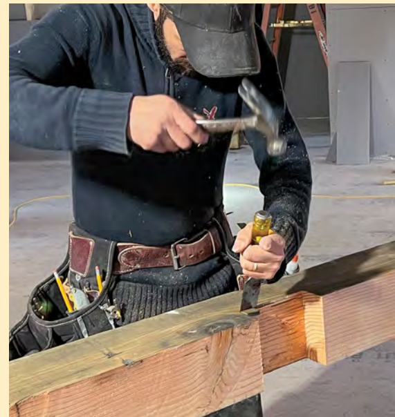
MORTISE CLEANOUT The beam is rotated onto its side and the waste is chiseled out from each side.
