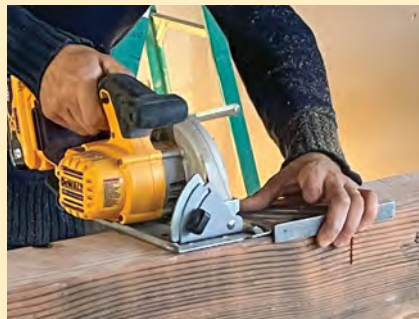
SQUARE SHOULDERS Cutting the mortises begins with circular-saw cuts across the beam to the depth of the joist tenons. A rafter square guides the cut to ensure the shoulders of the mortise are perfectly square. Additional cuts between the shoulders help with waste removal.
