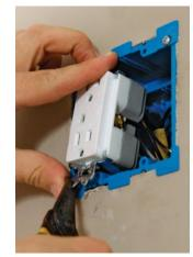
Break the ears for a flush fit. When installing receptacles in an old-work electrical box, slide the box into the hole in the wall to hold it securely while you work, but don't fasten it yet. When permanently installed, the grounded slot of the three-prong outlets should be on top. It helps to remove the "ears" from the receptacle to ensure a tight fit against the box so that the cover plate seats flat against the wall.
