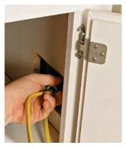
Conduit is faster than fish tape. After the holes have been drilled, snake the cable from the bracket hole to the temporary middle hole, then down into the cabinet. Insert a short run of conduit between the cabinet and the crawlspace, and snake the cable through it. Once the cable is in place, slide the conduit off like a sock.
