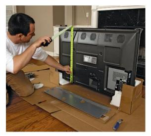
Leave the TV in the box. Use the cardboard packaging as a second pair of hands, and measure the height and width of the TV to determine the best location for the bracket to be mounted on the wall.
