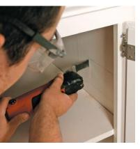
Careful cuts. A hole in the cabinet provides access to a nearby outlet or power in the crawlspace below and will later be used to connect A/V cables as well. Use an oscillating multitool or a small reciprocating saw for clean cuts in these tight quarters.
