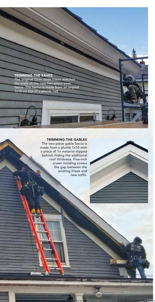
conceal the additional roof thickness. To get the overhangs straight and flat on this generally wonky roof, we used strings and shims to straighten the stock as we nailed it up, which took us a little longer than expected. With the battens and overhangs complete, we installed a layer of ½-in. plywood on top for the standing-seam roof.
