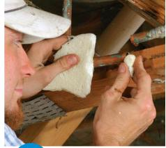
DAM THE DRIP A ball of white bread (photo above) stuffed inside piping will absorb trickling water. Once the water is turned back on, the bread should be purged from the plumbing via an exterior hose bib or a washingmachine-hose line. Plumber's bread (photo below) works the same way and won't become moldy in your plumbing kit.
