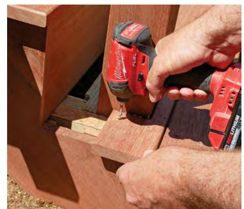
Avoid split ends. When screws are placed near the ends of the treads and the post notches, make sure to predrill pilot holes so that the boards won't split when fastened.
