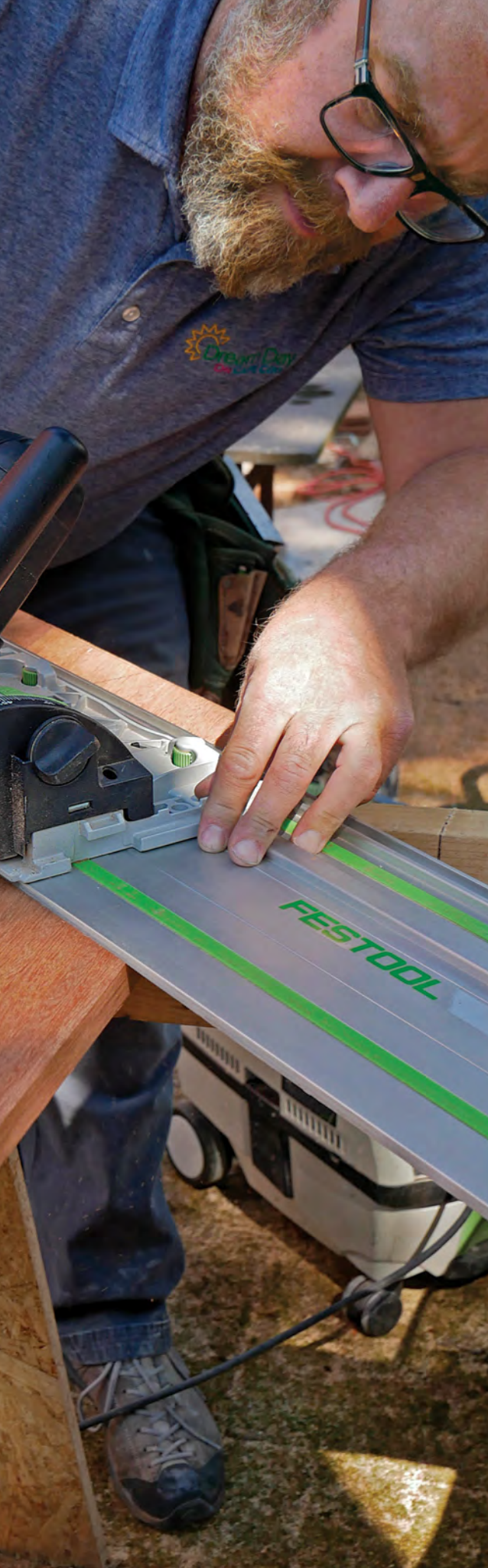
... then left. The other skirtboard's miter cuts require a saw that bevels to the left, which meant swapping the track saw for our miter saw.
