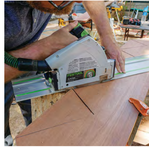
Add the straight cuts. Follow up the riser bevels by cutting the straight run lines (where the treads will land), and avoid overcutting.
