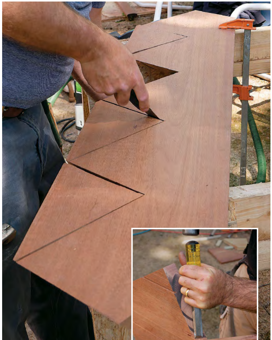
Finish and fine-tune the cuts. Use a pull saw to complete the cuts and a chisel to clean the corners.
