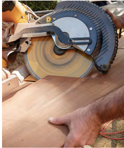
... then left. The other skirtboard's miter cuts require a saw that bevels to the left, which meant swapping the track saw for our miter saw.
