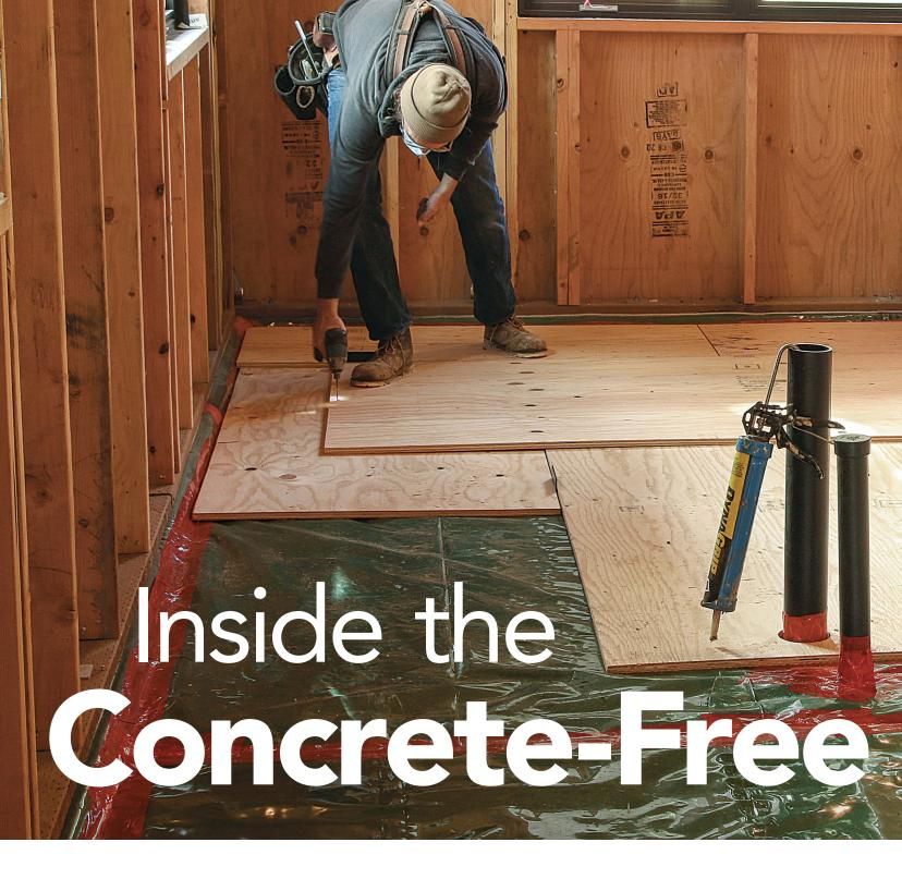
An innovative plywood slab-on-grade means less time, money, and carbon
