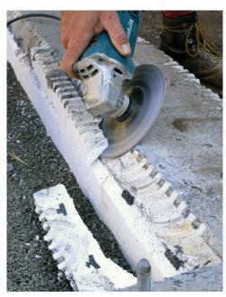
**BEVEL THE INSIDE EDGE OF THE FOAM** A 45° bevel makes it possible for the drywall and baseboard to cover the top of the foam at the edges of the floor.
