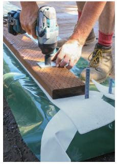
**VAPOR BARRIER UNDER THE SILL**The crew runs a strip of the vapor barrier under the sill plate before framing, later taping it to the interior vapor barrier.
