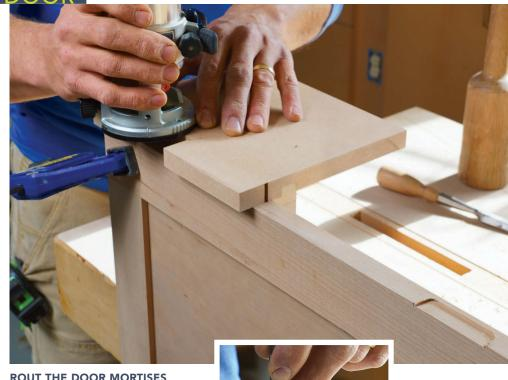
ROUT THE DOOR MORTISES To locate your router jig accurately on the knife lines, run a sharp pencil down each one to help it stand out.
