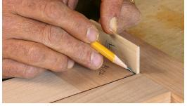
MARK THE TOP SIDE AND STRIKE SIDE Use the same shim-marking technique, being very careful to line up the outside of the shim with the inside of the face frame.
