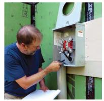
CHECK EXTERIOR PENETRATIONS Exhaust, dryer, and plumbing vents, electrical chases, and any parts of the heating and cooling system are likely spots for air-sealing before or after the test.
