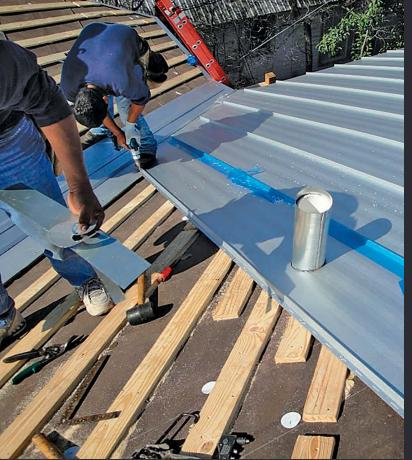
ridge cap—9 in. on each side. That allows air to come out the top, but rain can't get in.
