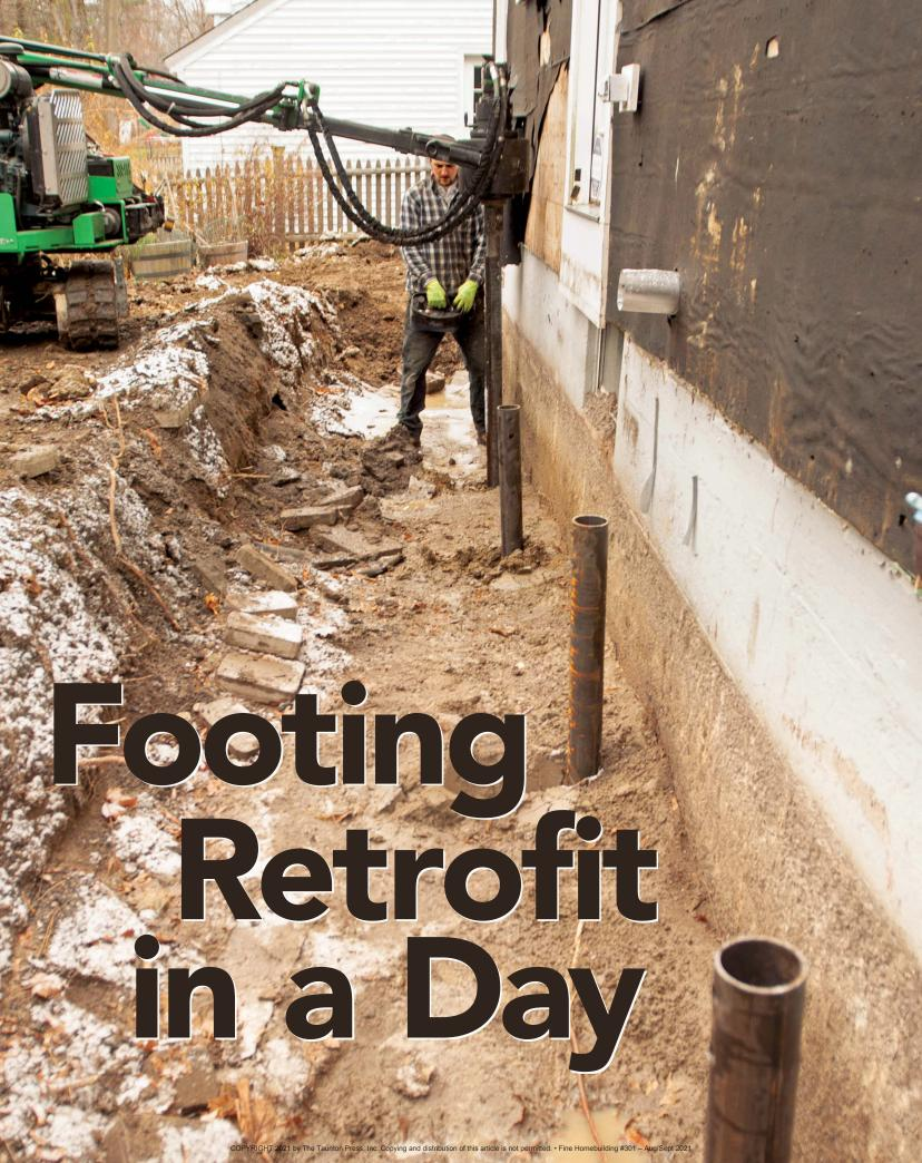
Using helical piers to add footings to an old house is faster, less disruptive, and comparable in cost to excavating and pouring concrete
