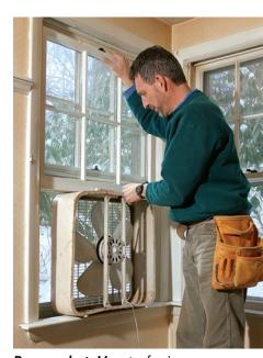
Remove dust. Mount a fan in the window to pull dust out of the house. Cover floor registers and return-air grilles. Furnace filters work well for this purpose if the heating system will be running during the job; otherwise, tape them shut with cardboard. electrical cable, pipe generally runs in a straight path, so it is fairly easy to sleuth out. Check in the basement for plumbing lines and in the attic for vent pipes.
