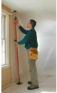
Contain dust. Clear plastic isolates the area without blocking light. Furring strips or telescoping poles (www.zipwall.com) hold it tight to the floor and ceiling. Protect your lungs with a respirator, and beware of lead paint. (For more on dust control, see FHB #180, pp. 78-83.)
