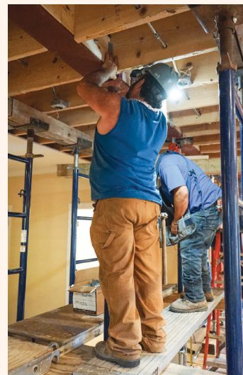
Secure the bases. Double-headed nails secure the post bases to the timbers that distribute the loads.
