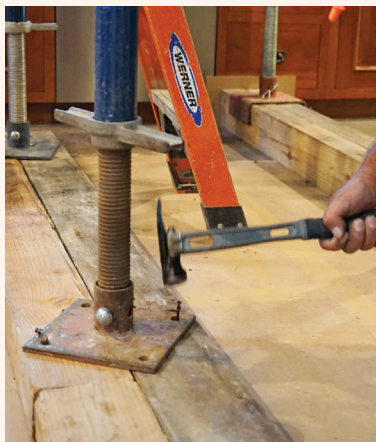
Secure the bases. Double-headed nails secure the post bases to the timbers that distribute the loads.
