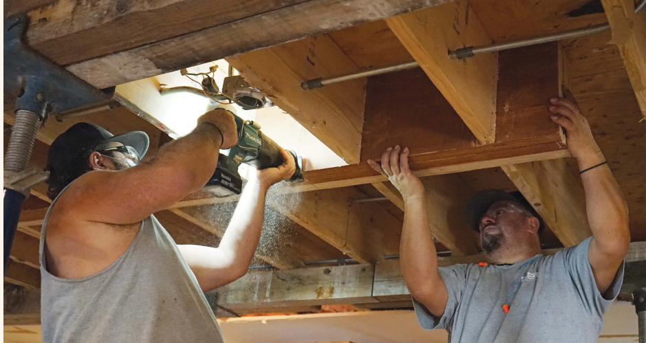
Failed-member removal. With the shoring in place and all the loads supported, the crew cuts the LVL beam into small pieces that are safer and easier to remove.
