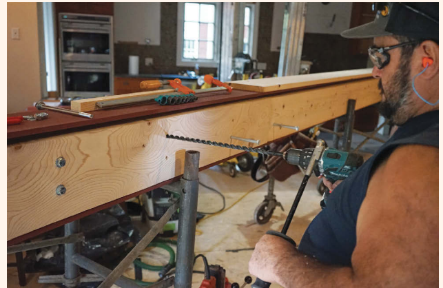
Proper sequencing. Sometimes the shoring can make it difficult to bring in the replacement structural element. Here the steel beam was put in position and prepped before the shoring was set up.
