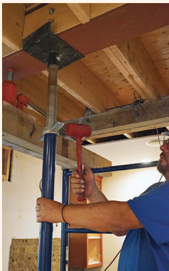
Secure the bases. Double-headed nails secure the post bases to the timbers that distribute the loads.
