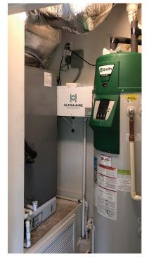
Systems can be small. Installers faced with a small mechanical room can still often squeeze a small high-capacity dehumidifier on a 2-ft. by 2-ft. wall section and connect it with flex duct. Compact models also exist for low-clearance attics and crawlspaces.
