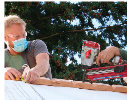
Horizontals go on first. One row of horizontal 2x4 nailers—with a series of V-notches cut in them to allow air to pass through—is installed at the ridge, and another at the eave.
