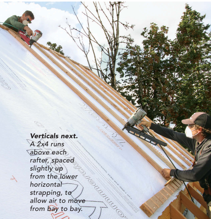
Roll out the WRB. A 10-ft.-wide roll of water-resistive barrier works perfectly with 24-in. rafter spacing. The team rolls it down or up, whichever is easier, and attaches it with staples.
