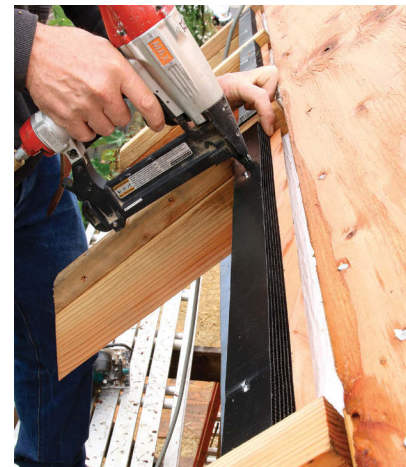
Insect-proof soffit vents. Cor-A-Vent S-400 soffit strips block insects and debris. At the 2x4 strapping that continues along the rafter tails, Breckenridge plywood will finish off the open-soffit design.
