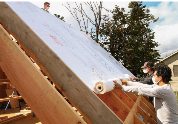
Roll out the WRB. A 10-ft.-wide roll of water-resistive barrier works perfectly with 24-in. rafter spacing. The team rolls it down or up, whichever is easier, and attaches it with staples.
