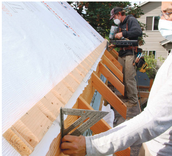
Horizontals go on first. One row of horizontal 2x4 nailers—with a series of V-notches cut in them to allow air to pass through—is installed at the ridge, and another at the eave.
