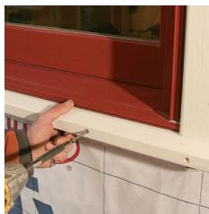
Sink the screwhead. Nail the head and legs every 9 in. using 2½-in. galvanized finish nails. Then screw the sill to the framing. Use a ¾-in. countersink bit to sink the screwhead about ½ in. below the surface. Fill the hole with a plug made of the same material.
