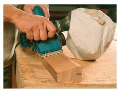
**Plane the face smooth.** Use a power planer to remove saw marks and to dimension the sill's flat top to equal the depth of the window's cladding.
