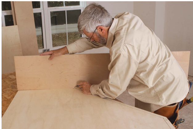
MARK IN PLACE When possible, use the layout lines as a guide to mark where to cut pieces to length.
