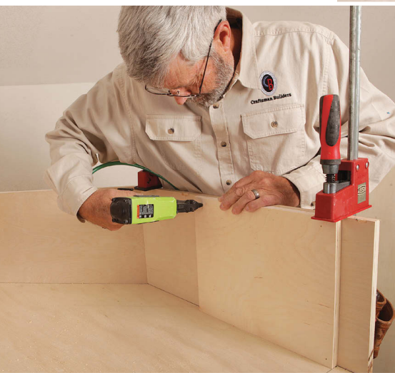
PREP THE POCKETS Pocket-hole screws secure the face frame along the sides that butt into the wall and ceiling. Drill the pocket holes before the entire perimeter of the cabinet is fastened to make things easier.
