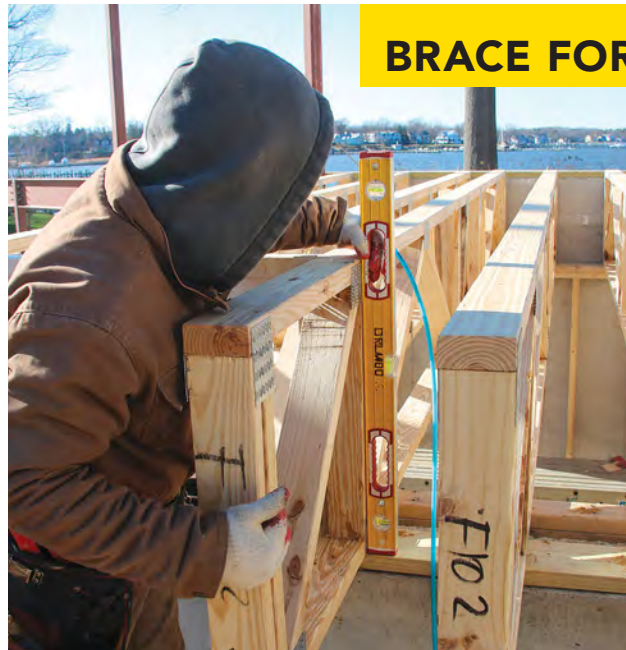
Check for plumb. These trusses, which overhang the foundation wall, will have 2x4 blocking cut to fit between the top chords above the foundation. We check pairs of neighboring trusses for plumb (and temporarily brace if necessary) so the blocking pieces are cut and installed at the correct length.
