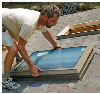
**The window, at last.** With the curb flashed and virtually watertight, I can fasten the window to the frame. This skylight was a fixed frame, so the counterflashing was part of the window frame. Don't forget to remove the protective plastic sheet before you descend the ladder.
