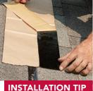
After I cut strips of self-adhesive membrane, I dry-fit them in place, then flip them over and score the release sheet along the fold line. Now I can stick the membrane to one surface and apply the other half when it's in place.
