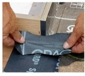
up this vulnerable area with small patch pieces of membrane 1½ in. to 2 in. wide. I make them bow-tie shaped so that they have more surface area that can bond to the skylight frame. I apply the strip firmly along one edge first, then stretch it through the corner before bonding to the other edge.
