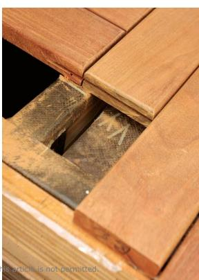
stainless-steel fasteners and take extra time installing them so that they looked like part of the design, a fascia board that hides the fasteners seemed like a logical option. This tack turned out to be of dubious economic value when compared with the price of stainless-steel fasteners, but it does dress things up.
