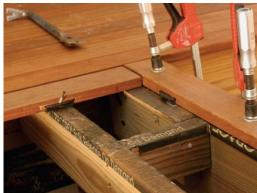
Slot the first board in place. After gluing and clamping the first board, determine where the second board will intersect and where the third board will end. Cut the slots using a router outfitted with a slot-cutting bit. Bending over the board to make a cut like this is dangerous, so use caution. Using a biscuit joiner before the board is installed is another option.
