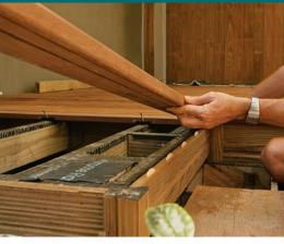
Biscuits replace screws. Instead of using screws and plugs through the face of the perimeter boards, the author chose to biscuit them to the fascia. Run the starter board long; it will be cut after the field is laid. Dry-fit the starter board with the biscuits in place. After applying glue to the biscuit slots, the biscuits, and the groove, reapply the board and clamp it in place.
