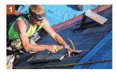
After every four or five courses of slate are installed, we nail a set of roof jacks to the rafters (1). The worst thing you can do to a slate roof is walk on it, because you will break slates. The rows of jacks are set close enough to get from one row of staging to another without stepping on the slate. Slating roof jacks are installed 8 ft. on center, with 1¾-in. by 9-in. LVL scaffold planks on top (2). It sounds like overkill, but at times the plank will hold piles of slates and two roofers.
