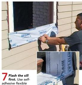
Flash the sill first. Use selfadhesive flexible flashing to create a waterproof sill pan. First, spread the
