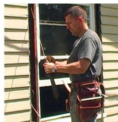
Weights, then window. After pulling out the loose sash weights, remove any fasteners holding the window in place, and lift the entire window frame from the opening in one piece.
