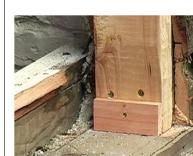
**5** Add blocking. Once the old window frame is removed, clear debris and errant nails. Use 2x lumber and spacers to block in the sash-weight cavity and to create the appropriately sized rough opening for the new window.
