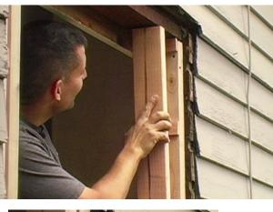
Fur out the blocking. The front face of the new rough opening should be flush with the sheathing. In this case, the author
