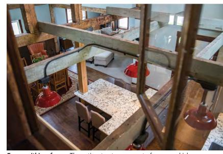
**Frame within a frame.** The entire structure was out of square, which was one of the reasons for rebuilding the gable-end walls. Originally, balloon-framed walls of native 2x4s, with studs spaced anywhere from 12 in. to 30 in. apart, capped the gable ends outboard of the timber frame. We removed those and replaced them with 2x6 walls for additional insulation and regular stud spacing.
