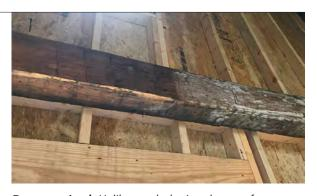
**Beams revived.** Unlike sand, dry ice changes from a solid to a gaseous state during the blasting process, producing microscopic shock waves that aid in cleaning the timber without damaging its character.
