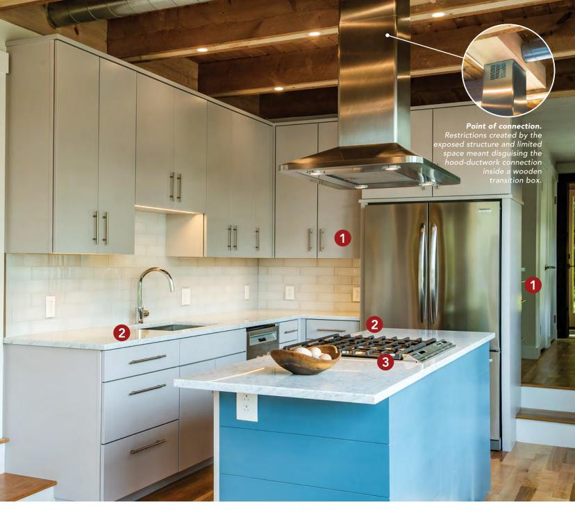
and floor. Task lighting includes the rangehood lights and high-output LED strip lights set into receiver tracks with frostedplastic diffusers under the upper cabinets. I'd never used that type of lighting over a sink, and I was worried that it might not provide enough light, but my clients are very happy with it.
