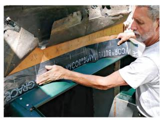
MANAGE WATER Apply self-adhered flashing tape over the header flange of the door, tucking it beneath the water-resistive barrier on the wall.
