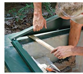
**BED THE FRAME** After applying sealant, slide out the shims one at a time and lower the frame, backfilling the areas where the shims were located with sealant.
