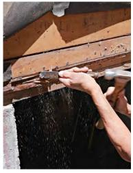
**TRIM THE SHEATHING** Use a circular saw with the blade set at the depth to be removed to cut along the flange mark, and follow up with a chisel to remove the remaining material to recess the flange.
