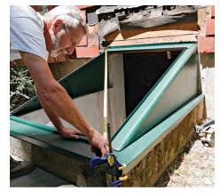
PLUMB AND SQUARE Dry-fit the door tight against the house and centered on the foundation plates. Measure diagonals to verify that the unit is square, adjusting as necessary.
