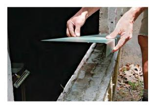
**INSTALL THE PLATES** Apply a thick bead of highquality sealant to the top of the clean foundation before installing the plates.
