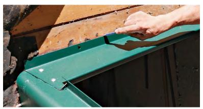
DRY-FIT THE FRAME Center the frame on the foundation and check the seal against the house. Here the 3/4-in. sheathing was about 3/8 in. proud of the concrete, so I traced the flange on the wall for a cutline.
