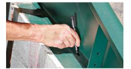
**PREPARE FOR DRILLING** Locate and mark the mounting holes on the foundation and walls.
