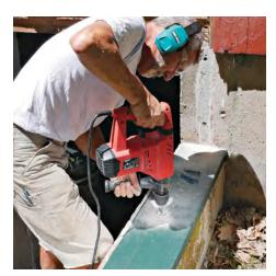
THROUGH THE METAL AND INTO THE MASONRY Start the holes in the foundation plates with a metal-drilling bit, then switch to a masonry drill and bit to finish boring through the thin remaining metal and into the concrete.
