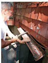
**DISASSEMBLE THE DOOR FRAME**After unbolting the sill and header sections from the side panels, remove the sill to free the side panels, fold the panels in toward the stair opening until they disengage, and then pry the header piece down from under the siding.
