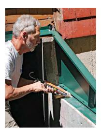
POSITION, SHIM, AND SEAL Shim the whole unit about 1 in. above the foundation and apply a bead of sealant along the foundation and walls for the new door frame to bed into.
