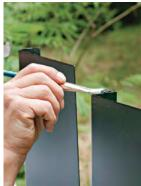
**CUT TO FIT** I cut the plates with a tungsten carbide metal-cutting blade in a circular saw; an angle grinder with a cutoff wheel can also be used. Prime and paint all cut edges.
