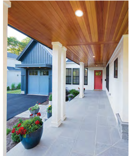
Elegant entry. The foundation was formed using a mudsill detail that has the joists slotted into, rather than on top of, the foundation, meaning the house sits low to the ground. This profile helps accentuate the front porch.
