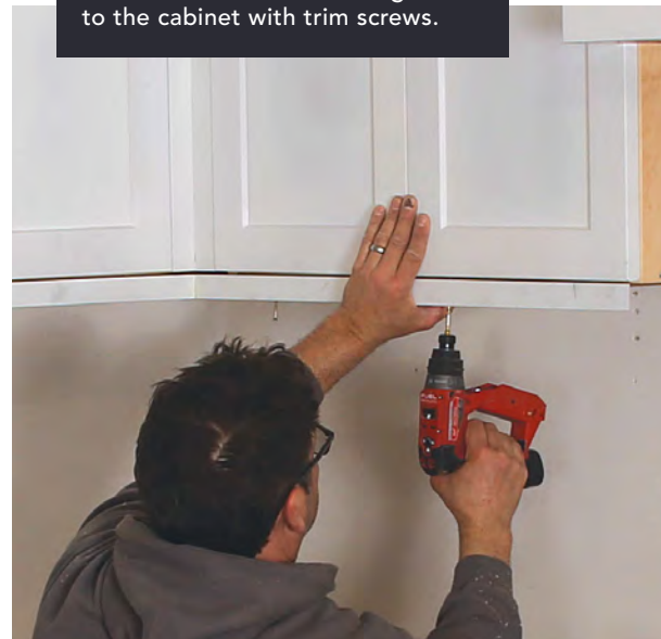
LIGHT RAIL LAST Joints are coated with wood glue and a squirt of CA glue for a quick bond. Once assembled, we attach the light rail to the cabinet with trim screws.
