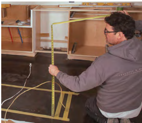
LASER CHECK We set up a laser level and measure up to it in multiple places on the island's perimeter to determine if there are high spots that require trimming the cabinet bottoms to keep them in plane with the lower cabinets.
