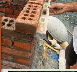
Gauge the corbel. To dress up the top of the chimney, I like to step out the brick into what's called a corbel. Each brick should overhang around 3/8 in. to 1/2 in. Any more, and there won't be an adequate connection to the underlying course. I use the white ovals surrounding the bubble on my level as a gauge.
