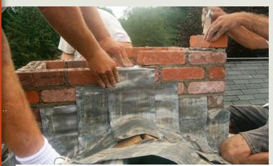
Leave the lead long. The apron flashing should cover the entire lower face of the chimney and wrap a few inches around the corners, where it will be covered by the side cap flashing. To lock the flashing in place, use the point of a trowel to push the soft lead into the holes in the brick. Once cured, the mortar joint will hold the lead tightly. The flashing needs to be folded back when the roofing underlayment is installed, so leave plenty of extra flashing material to work with.
