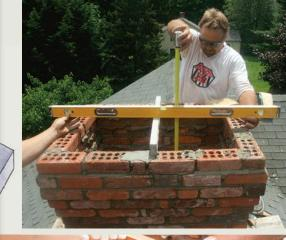
Stack levels to find the flue height. To find the height of the last section of flue tiles, which are sold in 2-ft. lengths, lay one level across the chimney opening to represent the rough height of the finished chimney crown, typically 2 in. or so. Then lay a second level perpendicular to the first to gauge the height that the new flue tile will extend past the crown, typically about 3 in. Finally, cut the flue tile to size using an angle grinder.
