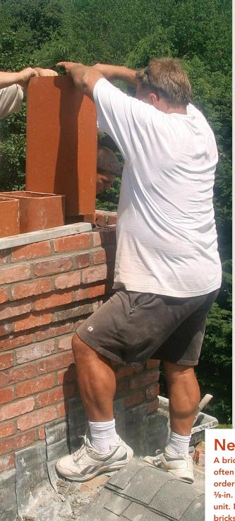
Scraps become the base for the crown. Fill the empty space between the bricks and the flue tiles with scrap bricks and mortar as you work. Lay the flat sections of an old flue tile across the top of the chimney in a bed of mortar.
