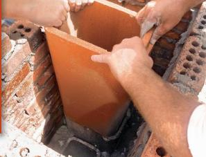
Flue mortar must be smoothed. Clean up the top edge of the existing flue tiles with a stiff-bristle brush, add a healthy dose of mortar, and then lower the new flues into place. Rough, ragged mortar joints can lead to dangerous creosote buildup. Reach down inside the flue tiles, and make sure that the gap is mortared fully. Then smooth it out with your hand.
