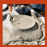
When it's time to rebuild, mix a batch of mortar, but don't wing it on this step. Mixing mortar is all about consistency. I mix my own batches on site using sand, cement, and water, but you can also buy mortar mix that just requires water. I combine one 80-lb. bag of type-S cement, three 5-gal. buckets of fine sand, and 3½ gal. to 4 gal. of clean water. If mixing by hand, I cut the quantities in half. The mortar should look smooth and fluffy.
