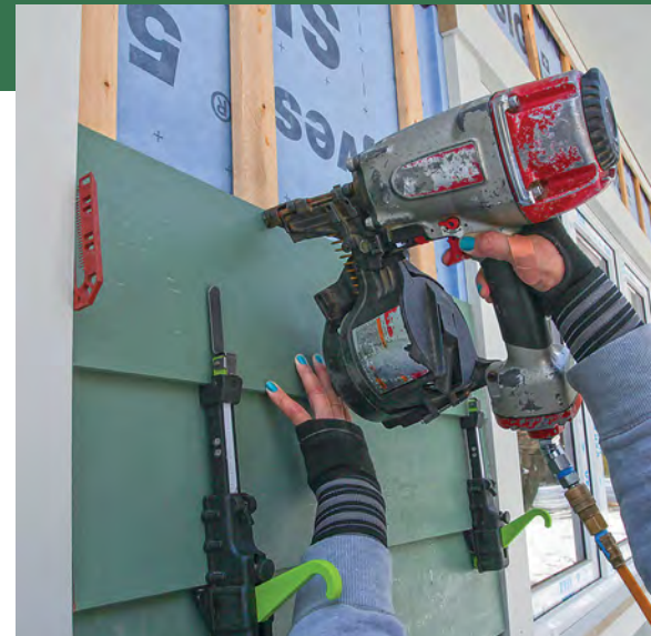
Leveled out. Check for level periodically to ensure everything stays on track. The siding gauges should keep everything parallel, but slight mistakes can easily compound if not caught.
