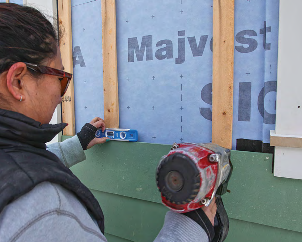
Leveled out. Check for level periodically to ensure everything stays on track. The siding gauges should keep everything parallel, but slight mistakes can easily compound if not caught.
