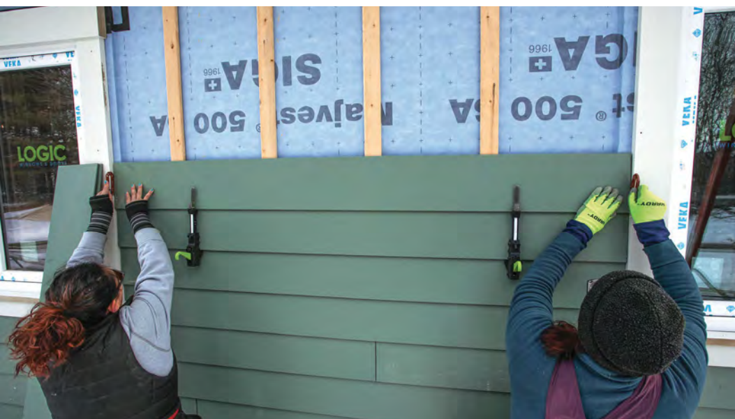
Mind the gap. Use \frac{3}{16} -in. shims to check the gap on both ends before nailing. Use the same shims to gap butt joints between pieces of siding.
