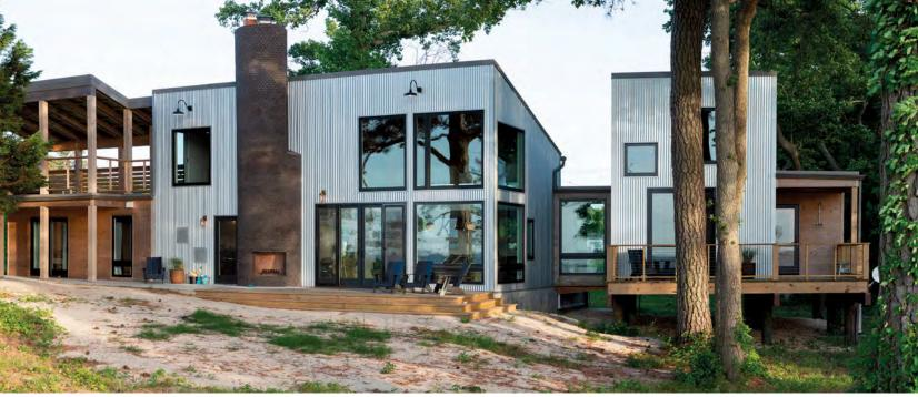
Rear in steel. Because the windows are concentrated on the back side of the house, which faces the water and is vulnerable to strong northwest winds, the engineers recommended steel framing. Wrapping the SIPs around structural steel presented a challenge that the builder resolved by welding bolts to the beams and then bolting 2xs to them. To avoid penetrating SIPs, the steel beam in the roof plate was stopped just short of the exterior wall and made to bear on a metal post.
