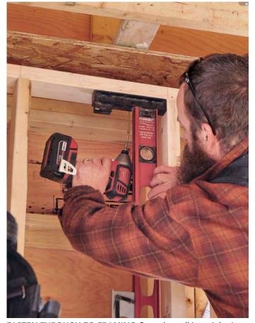
FASTEN THROUGH TO FRAMING Once the wall is upright, it has to be plumbed in both directions before being fastened. We use screws driven through the top plate and into the flange above, which should already be backed up by the ceiling framing.
