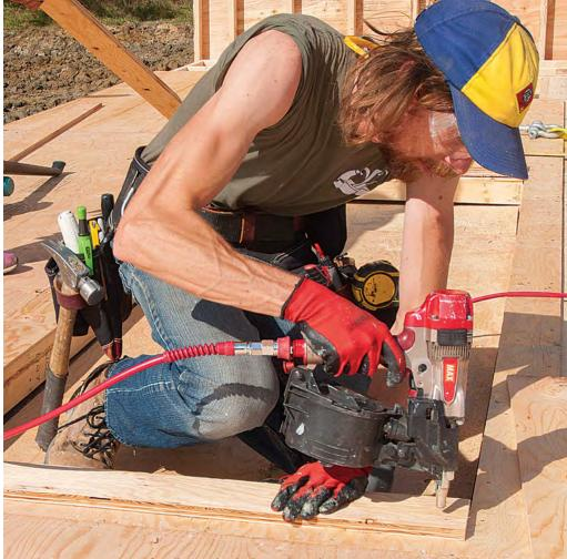
WHY PLY We prefer plywood, which is relatively vapor-open compared to OSB options, to allow the wall assembly to dry to the exterior. We pad out window and door openings to match the thickness of the rainscreen before installing the self-adhering WRB, making it easier to integrate the window flashing later.
