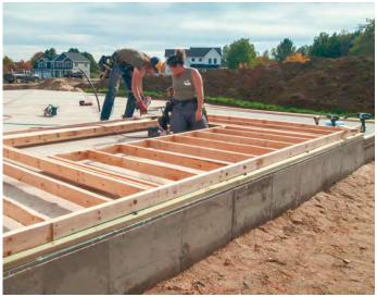
**OUTER WALLS ARE EASY** We rely on the outer walls to carry the loads of the structure, but since there isn't much concern about limited cavity insulation or thermal bridging, we use 2x4s and space them at the conventional 16-in. layout.
