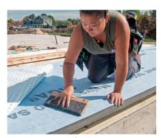
**LET IT BREATHE** The vapor-open nature of plywood only helps if you choose a vapor-open WRB and provide ventilation between the WRB and the cladding.
