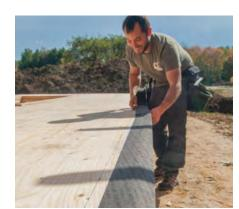
THINK AHEAD Split-release airsealing tape is a clean and effective way to connect the wall framing to the foundation below. Apply it before the WRB and rainscreen system are installed, overhanging it to be adhered to the concrete after the wall is tipped into place.
