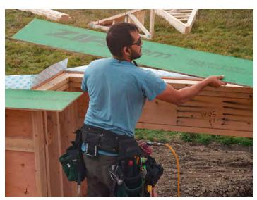
**CAP THE WALL** To connect the inner and outer walls and maintain the continuity of the air barrier, we install strips of sheathing to the outer-wall top plates, overhanging toward the inside. The flanges should be a few inches wider than the total wall thickness.
