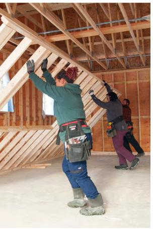
ROOM TO RAISE To make the inner stud wall easy to tip into place, we frame it 1½ in. shorter than the exterior—easy to do by simply using one less plate than the exterior wall.
