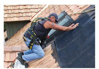
More matrix. Once the shingle courses have reached the top of the ventilation matrix, another row of matrix is butted to the previous course and fastened with stainless staples. Tuck the matrix under step flashing, lap it onto valley flashing, then cut with a utility knife.
