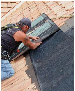
Flashing pipes and penetrations on a cedar-shake roof is similar to flashing asphalt and slate roofs—layers are lapped from the bottom up. Sidewalls get step flashing at every row; wider shakes are used at the wall-to-roof intersection. Headwall details get standard aprons.
