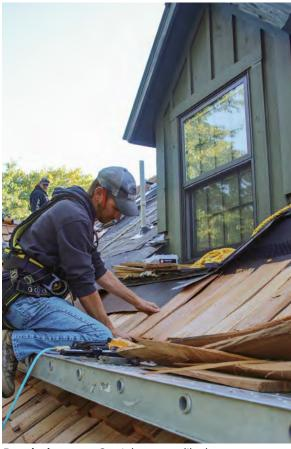
Rough character. On tight spaces like between this dormer and a neighboring valley, it often takes more than one try to get an arrangement of shakes that provides the minimum offset, maintains the saw-tooth pattern, and has a pleasing look.
