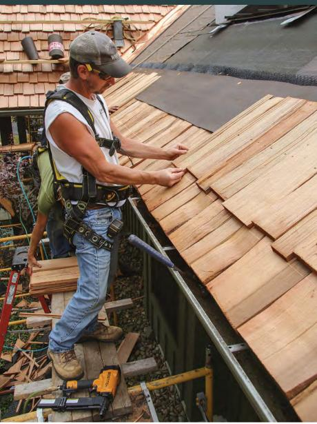
Whole lotta shakin' goin' on. Roofers work from both ends of the course and meet in the middle. Keeping a mix of shake widths close by helps ensure correct overlaps and an aesthetically pleasing layout.
