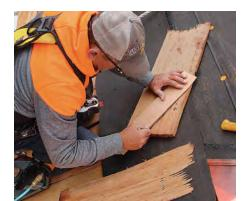
Scribe to fit. Use a scrap of shingle ripped to  $2^{1}/2$  in. as a guide for the angled cuts adjacent to the valley. This ensures that the cuts are straight and the sides of the valley are parallel from top to bottom.
