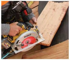
Cut on the roof. A cordless circular saw is the fastest way to make straight and angled cuts. For best results, rest the end of the shake on the roof to steady the piece while it's being cut.
