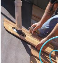
Flashing pipes. For the vent stack, place the boot on the ventilation matrix with the downslope edge lapped over the felt and shingle course below. A single shake with a round cutout is then fastened on top. A cordless jigsaw is the perfect tool for cutting the hole.
