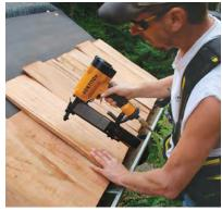
Finally, the first course. The first row of shakes lines up with the starter course below. Each shake is fastened with two stainless-steel staples 3/4 in. from the edges and 11/2 in. above the exposure line. Shakes should be spaced 3/8 in. to 5/8 in. apart with joints offset by at least 11/2 in.
