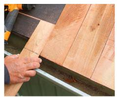
Starters before shakes. Under the first course of shakes is a starter course of underlayment shingles that overhang the fascia 1½ in. (rake ends overhang 1 in.). These are sawn, 18-in.-long., ½-in.-thick (at the butt) cedar shingles. Their thinner butt end keeps the first row of shakes from flaring up.
