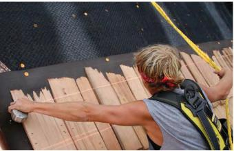
**Snap some lines.** The courses of felt and shakes are indicated by three snapped lines. The top one is for the felt interlacing; the bottom two indicate the exposure, which for this roof's saw-tooth design alternates between 9 in. and 10 in.
