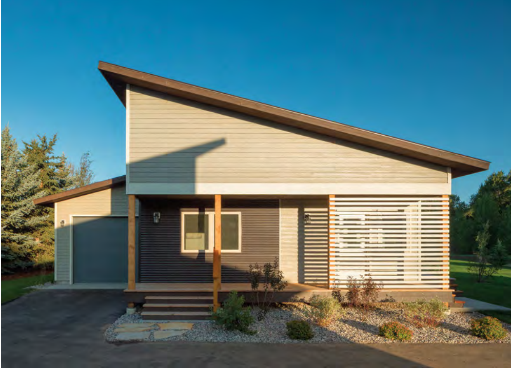
Base plan. This semi-custom structure features key components of all six houses. Each has a shed roof, an attached garage, wood screening, a combination of metal and clapboard siding, drought-tolerant foundation plantings, and at least one outdoor living space.
