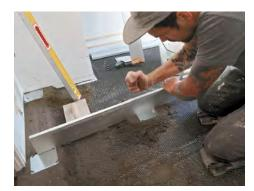
ADD A GO-BETWEEN Set a long screed between rows 1 and 2 so that an intermediate pier can be established in line with the outside corner of the bumpout (photo above). This pier will be used to establish rows 4 and 5 (photo right).
