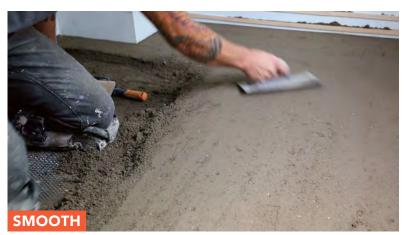
Last, slick down the top layer with a finishing trowel. This embeds the loose sand and brings a small amount of water to the surface, creating a thin crust that acts as a temporary wear layer until the floor is tiled.
