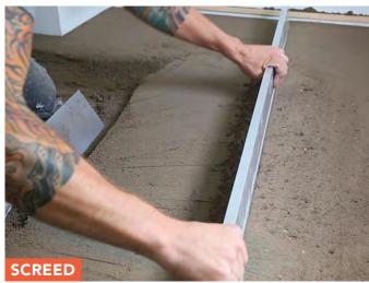
Pull a screed across the mud using a back-and-forth sawing motion, but don't let the ends of the screed dig in. After the first pass, use longer strokes to smooth the surface.
