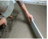
VOIDS If any areas have small holes or a piece of aggregate has created a divot, you can forcefully throw a handful of sand into the top layer of your mud. This embeds the sand particles into the mud and again ensures that you do not have a false bond that may separate when curing. Follow up by burnishing the surface with your wood float again.
