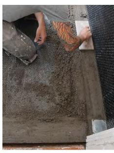
MAKE A CONNECTION Establish row 3, along the edge of the tub, to connect rows 1 and 2. This new row will then make it possible to create row 4.
