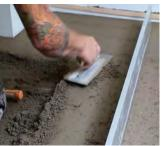
LOW SPOTS If you notice that any areas need additional material, rake the area loose, add more mud, re-pack it, and re-screed it. If you were to add material to the compressed mud without raking it loose, it would be compacted in separate lifts, and would create a false bond that could lift or separate while curing.
