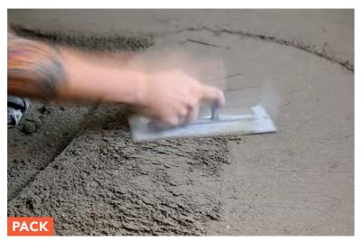
Using a finishing trowel, slap the mud with a firm, even pressure across every square inch. This hand pressure compacts the mud into a cohesive slab, hence the name "dry pack."
