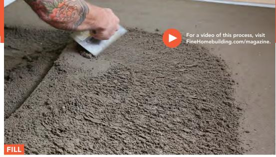
I aim to spread the mix roughly  $\frac{1}{2}$  in. to  $\frac{3}{4}$  in. higher than the existing screeds to ensure that once packed, it's not too low. Do not spread more mix than you can comfortably reach across and spread; my sweet spot is 16-in.- to 24-in.-wide sections.
