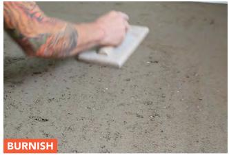
After screeding, use a wood float to burnish the top layer. The square edges get rid of any highs and lows in your bed, and rubbing in a circular motion fills any small voids.
