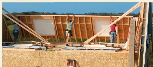
Raise the wall, but not quite plumb. Unless ceiling joists will bear directly on the top plate of the front wall, I like to lean the wall in about ½ in. before bracing it; the rafter loads will push the wall out as the building settles and the crowns on the rafters flatten.
