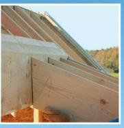
With a little extra planning, all the dormer components fit together nicely on the first try. For instance, the full-size drawing made it obvious that to ensure a smooth transition between the two different planes of roof sheathing, the dormer rafters (photo left) should be cut so that they sit just below the beveled dormer header.
