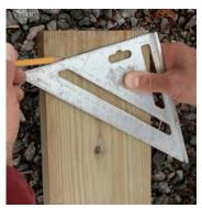
Figure out post lengths. Mark and cut the tops of the front and rear posts to match the height and pitch of the roof. If you did an accurate drawing, you should be able to pull the lengths and cut angles right from it, but you can also lay the posts out on the ground with a sill beam, a rafter, and a tape measure and mark your cuts in place.
