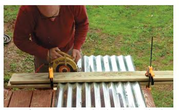
**Cutting sheets on-site.** Clamp a board or other straight edge onto the entire stack of panels and use a metal-cutting blade in a circular saw to make quick and clean cuts in the roof panels.
