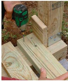
Fasten floor boards. Attach the 2x4s at the front and back, putting two 3-in. screws into the boards where they cross each beam. Infill with enough floor boards to leave 1-in. gaps for airflow to help dry the firewood. Use 1-in.-thick scraps to space them out as you fasten them down.
