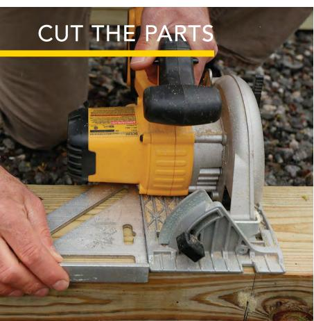
**Cut floor beams to length.** The shed depth and resulting beam length are based on how many courses of firewood you want to fit in the shed—in this case, three. Consider the proportions that will look good and use a common board length that will leave little waste after being cut to size. Make two passes with a circular saw for the cuts.
