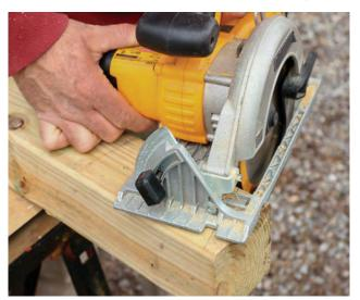
**Cut posts.** Flush-mounted rafters are held in place with TimberLok screws because the rafters are just supporting a lightweight metal roof. If this method won't pass code where you live, mark and cut 1½-in. notches at the tops of the posts.
