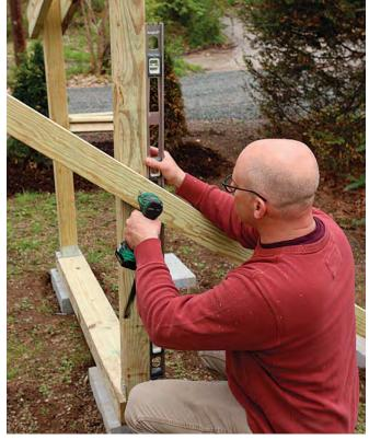
**Plumb the posts.** Attach temporary diagonal bracing to keep the shed frame plumb and square until there are enough floor and wall boards attached to lock everything in place. Keep the bracing completely inside the perimeter of the shed on the back posts so it won't be in the way when installing the walls.
