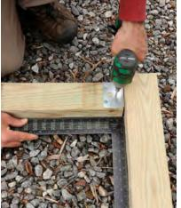
In hindsight... You will attach the posts while the sill beams are lying on their sides, so learn from my mistake and orient the hardware so the fastening flanges are on the front and back instead of the sides—otherwise you will have to flip the whole assembly over to drive the screws on one side of the base.
