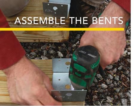
**Attach post bases.** Fasten the bases to the ends of the beams. Put them all the way to the edge for the side beams and center the hardware on the center beam. To keep things simple, these post bases are installed with screws rather than bolts.
