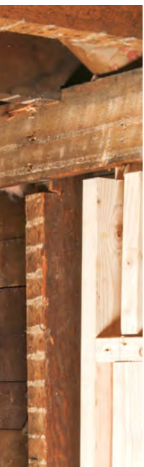
Cut the ribbon. Use a reciprocating saw to cut the old ribbon board on both ends and then use a cat's paw to remove the nails that hold it to the studs.
