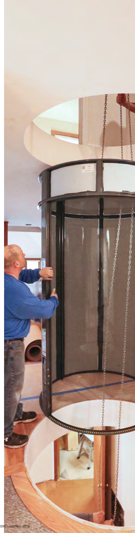
Starting point. Two crew members are stationed on the basement floor, two on the first, and one on the second to feed the tube sections up one at a time.
