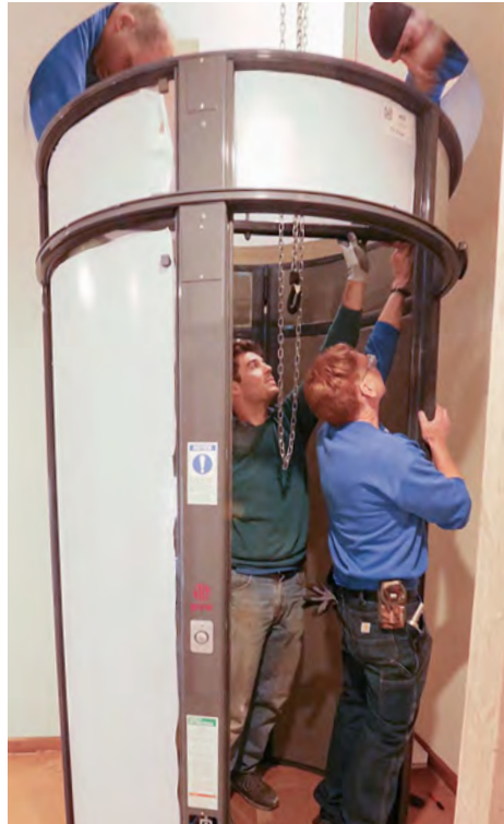
Starting point. Two crew members are stationed on the basement floor, two on the first, and one on the second to feed the tube sections up one at a time.
