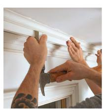
Drive to the line. Use a hammer and beater block to nudge moldings to their marks. This technique works even better with the bed molding than with the cove.
