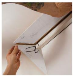
**Reinforce miters.** Biscuit every miter in the soffit, and cut the slots closer to the edge that faces into the room. Glue both slots and the faces of the miters before assembling.
