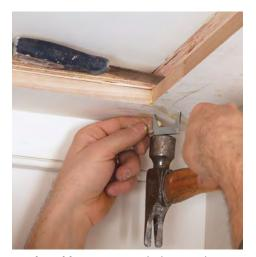
**Pinch and lever.** Use pinch dogs to draw miters tight where traditional clamps can't reach. A stiff putty knife is useful to adjust pieces into plane and hold them there while hammering in pinch dogs or nailing.
