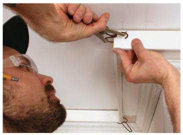
Clamp inside and out. Use wood glue and pinch clamps on both outside and, because they're accessible, inside miters.
