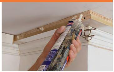
Dab glue. Apply dabs of PL glue every 12 in. to bolster the fascia's connection to the rest of the assembly.
