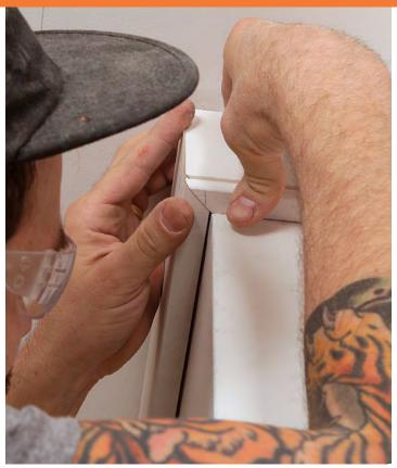
**Line it up.** Dry-fit joints before fastening the pieces. This often requires having the pieces they intersect at the far ends either installed or dry-fit to ensure the lengths and miters are spot on. A helper or two is required for this step.
