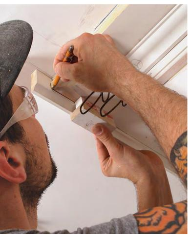
Gauge and mark. Use an L-shaped gauge block set to the reveal below the soffit to establish the height of the fascia, and mark the reveal and the outside miter cut at the same time.
