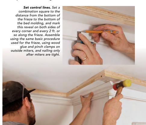
**Drive to fit.** Use a soft hammer to coax inside miters tight before marking the cut for an outside miter and fastening the free end of the intersecting piece.
