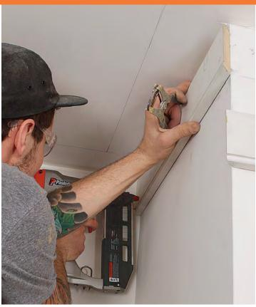
**Fastened but free.** Apply beads of polyurethane adhesive to the back of the piece and to the coped joint to provide reinforcement. Don't fasten the mitered end to the wall until that joint is assembled.
