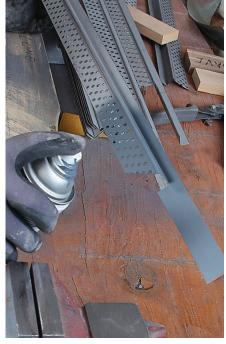
**Prime cuts.** Spray cut pieces with gray primer so you can see the joints better when dry-fitting miters and transitions. The primer also makes the installation look more finished.
