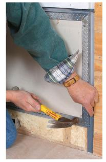
**Nail it up.** In addition to construction adhesive, the reglet trim is held with ring-shank nails made for exterior stucco trims like weep screed and outside corners. They have a thicker shank and deeper rings than drywall nails.
