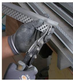
**Use snips for small cuts.** Highquality aviation snips also work for cuts. Wear gloves when handling the pieces because even the factory-cut edges are razor sharp.
