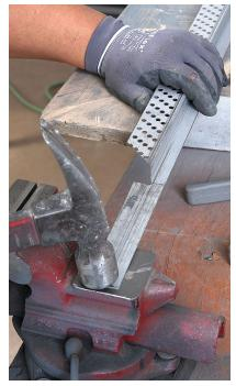
**Metalwork.** A small bench vice, a smooth-faced hammer, and hand benders help with fabrication. This piece of reglet intersects with a piece of base trim; we flatten the "L" so the poplar base can overlap without gaps.
