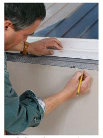
**Dry-fit first.** After cutting, dryfit the reglet parts using drywall screws to temporarily hold them in place. Adjust the fit until all the miters are tight and then mark the inside perimeter to guide the placement of construction adhesive.
