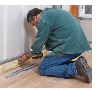
**Case, then base.** Once the window trim is complete, we install the trim for adjacent baseboard. When all the reglet is in place, we sand and finish the hardwood floors before the baseboard is installed.
