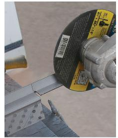
**Use a grinder for rip cuts.** An angle grinder with a steel-cutting abrasive blade is best for removing flanges and making stopped cuts. Remove burrs with a file or wire brush so joints are tight.
