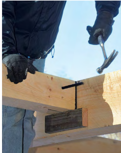
Install the 6x6 joists. To support the overhead storage loft, install three 6x6 joists similarly to the crossbeams. Screw the connectors flush to the tops of the crossbeams before installing the 2x4 joist-support cleats. With the 6x6 joists in place, drive two pins through each end of each joist.
