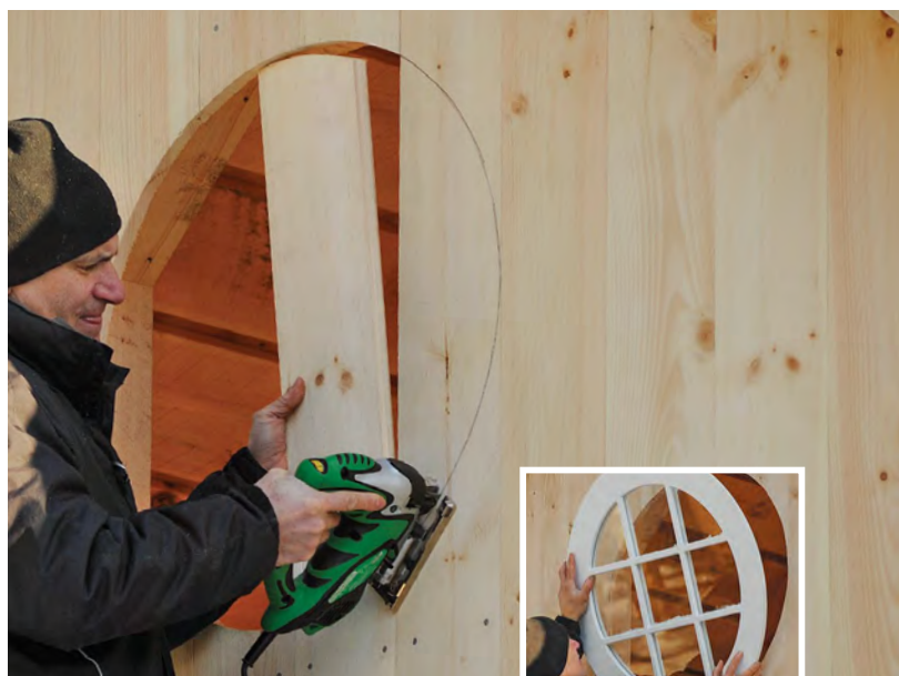
Cut the circle. When framing the round window, space two posts slightly more than the window diameter apart, and fill in the corners with angled nailers. After the siding is up, attach a string to a screw in the opening's centerpoint, and tie a pencil to the other end. Use it to draw a 30-in.-dia. circle onto the siding, and then cut out the opening with a jigsaw.
