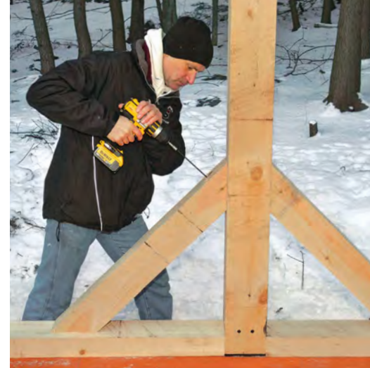
Brace the frame. With the beams in place, secure the 4x6 bottom plate and the 4x5 wall braces with 8-in. structural screws, drilling deep counterbores so the holes can be plugged for a clean look. Then add nailers and blocking for windows, doors, and siding.
