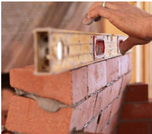
Top it off. Custom-cut and lay the last course of the firebox's back wall level and plumb to carry the damper. Lay sidewall bricks as necessary to stabilize the curve, but leave space for the lintel, and fill in the sidewalls level with the back wall after the lintel is set.
