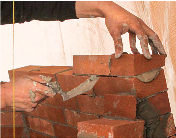
Top it off. Custom-cut and lay the last course of the firebox's back wall level and plumb to carry the damper. Lay sidewall bricks as necessary to stabilize the curve, but leave space for the lintel, and fill in the sidewalls level with the back wall after the lintel is set.
