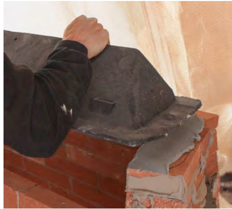
Set the damper. Remove the damper's flap to make it easier to handle and set it atop the firebox.
