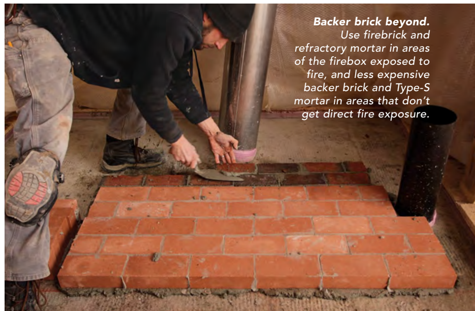
Stay on bond. Mark the center of a brick in the preceding course to help keep the bond pattern perfect. Keep joints tight at about \frac{1}{16} in.
