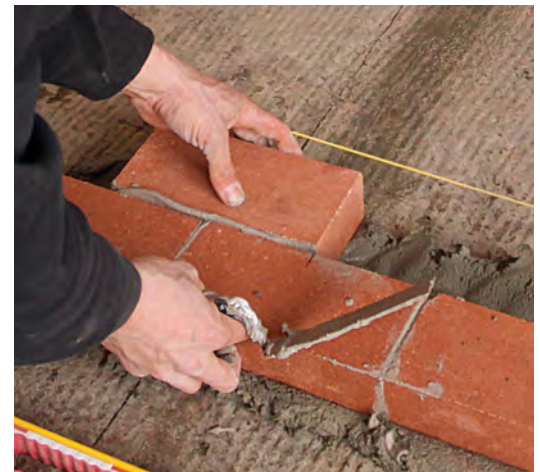
Stay on bond. Mark the center of a brick in the preceding course to help keep the bond pattern perfect. Keep joints tight at about \frac{1}{16} in.
