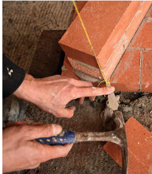
String for plumb. Use stringlines where possible. Here, stringlines plumbed down from a temporary outrigger aid in laying the front edge of the sidewalls plumb. Screws hold the lines in place above, and line pins secure them under the first course of bricks.
