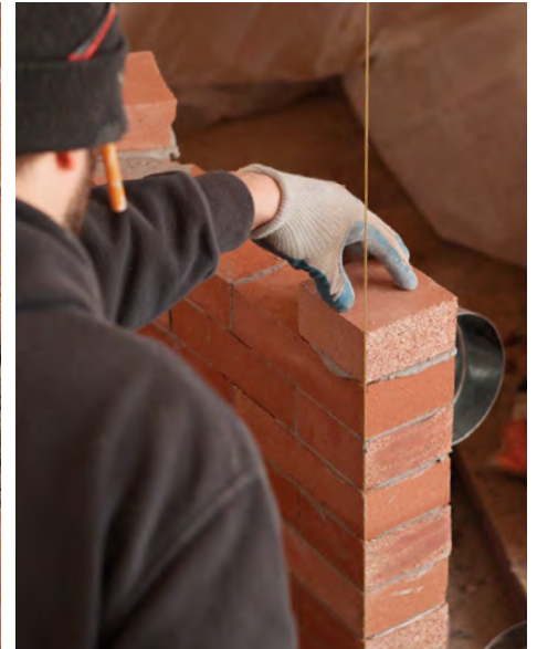
String for plumb. Use stringlines where possible. Here, stringlines plumbed down from a temporary outrigger aid in laying the front edge of the sidewalls plumb. Screws hold the lines in place above, and line pins secure them under the first course of bricks.
