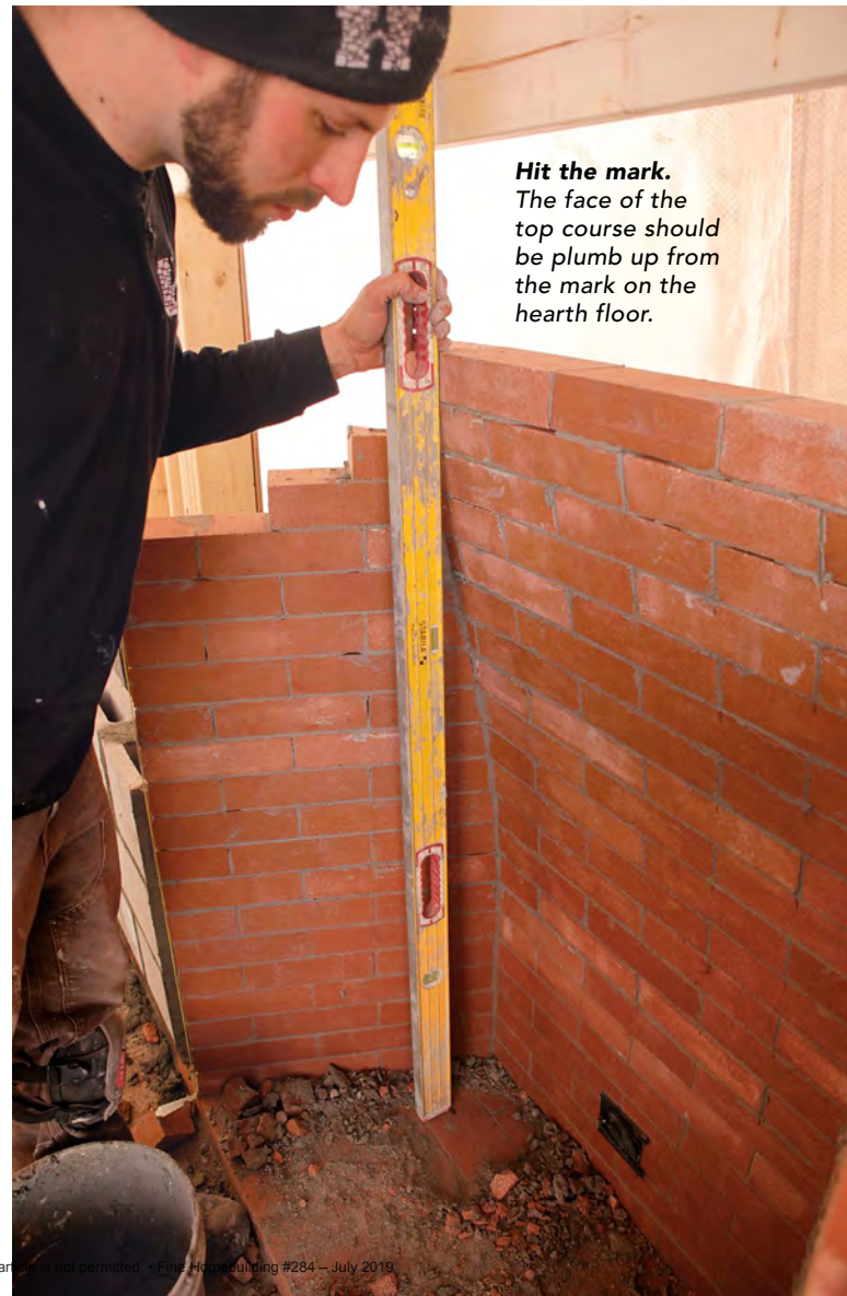
Stop the curve. Use a level and a tape measure to determine how much needs to be trimmed from the bottom of the last course of bricks to level the back wall.
