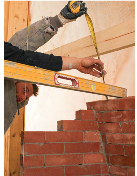
Stop the curve. Use a level and a tape measure to determine how much needs to be trimmed from the bottom of the last course of bricks to level the back wall.
