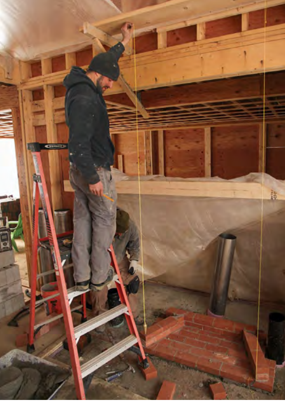
String for plumb. Use stringlines where possible. Here, stringlines plumbed down from a temporary outrigger aid in laying the front edge of the sidewalls plumb. Screws hold the lines in place above, and line pins secure them under the first course of bricks.
