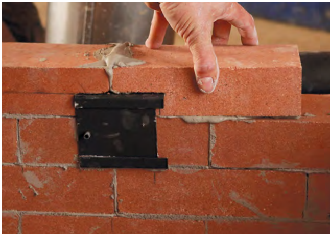
Get some air. If makeup air isn't supplied to a room mechanically, supply vents are required in the firebox. Follow the manufacturer's instructions for supply-vent installation.
