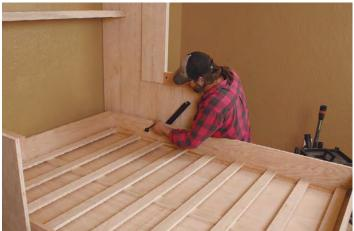
Connect the bed to its cabinet. The bed box is connected to the hinges with large-shouldered through bolts (included with the kit) that are tightened with a 10-mm hex wrench. Most hexkey assortments don't include a wrench that big, but you can find them at auto-parts stores.
