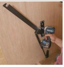
Mount the hardware. The hinges and lift supports are bolted to the bed cabinet's sides using locking nuts and through bolts. Gas pistons help balance the weight of the bed box and the mattress. The pistons are matched to the bed size.
