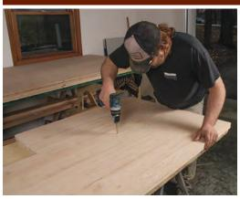
Double drilling. The hinge and lift mechanisms require identical holes for through bolts on both sides of the cabinets. It's faster and more accurate to drill both sides at once. Triple-check their locations so that the mechanisms work correctly when the desk bed is complete.
