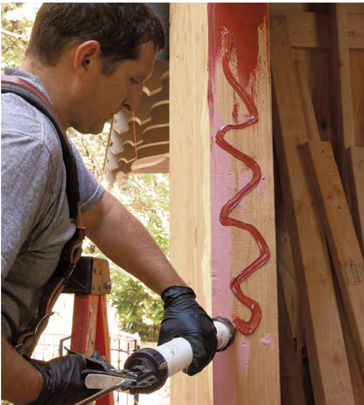
Coat the inside. FastFlash must extend inside the rough opening at least 1 in. past the window jamb. These windows have extension jambs that cover the full stud, so all of the jack stud is covered.
