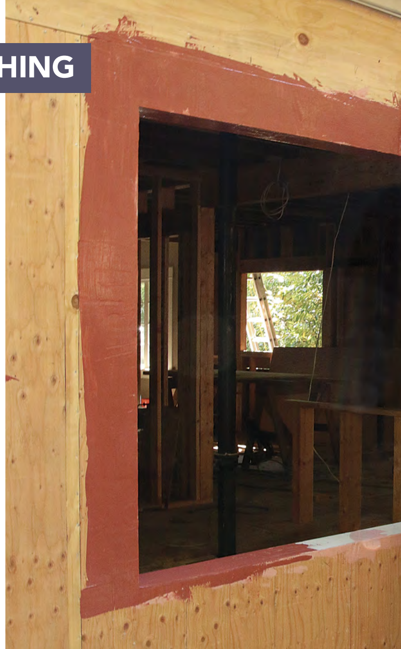
Coat the inside. FastFlash must extend inside the rough opening at least 1 in. past the window jamb. These windows have extension jambs that cover the full stud, so all of the jack stud is covered.
