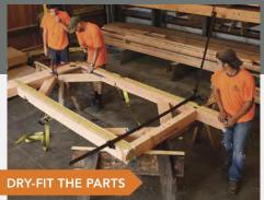
Once all the components are ready, individual frame sections are assembled and made square with pipe clamps, ratchet straps, and dead-blow hammers. Sturdy sawhorses put the parts at a comfortable working height.
