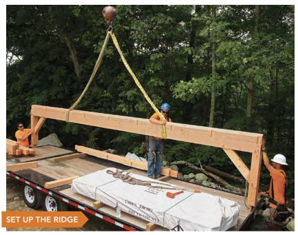
Before lifting the ridge beam into place, the short posts it bears on and reinforcing braces are assembled on the delivery trailer. Whenever possible, roof components are assembled on the ground to minimize working at height.
