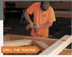
Once the pieces are together and square, the framers drill holes through the tenons using the machine-cut holes in the mortises as a guide. The pieces are then taken apart, banded, and placed on pallets for delivery.
