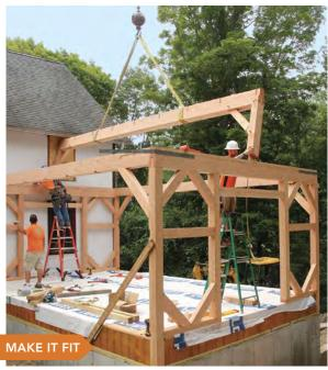
The roof of this timber-frame addition tucks under the eave of the existing building. The ridge height was planned to leave enough room to fit 2x6 tongue-and-groove sheathing and shingles under the eave.
