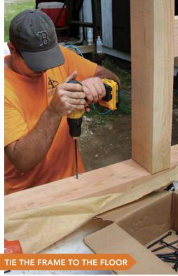
The final step is to drive structural screws to connect the frame's bottom plate to the LVL band joist. This step helps to control uplift during high winds. Predrilling prevents splitting the LVL.
